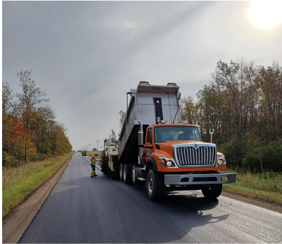
Paving on CTH WW rehabilitation project
