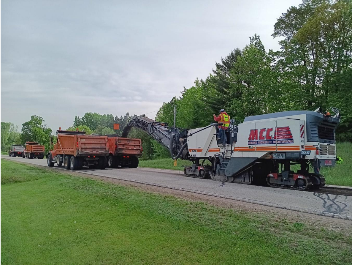
Milling on CTH BB rehabilitation project
