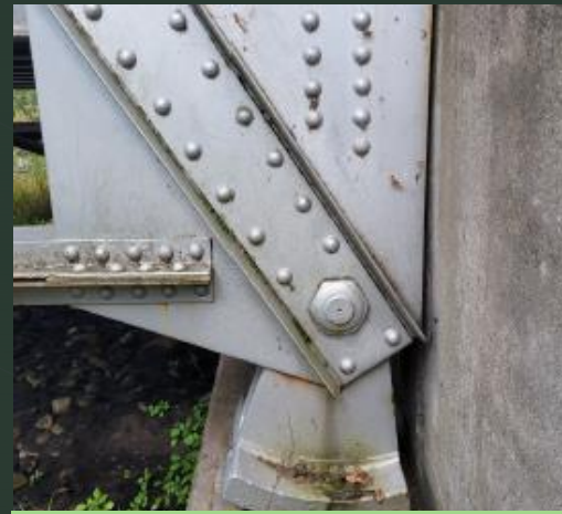
East Expansion Bearings.
