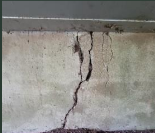
East Abutment – Vertical Crack.
