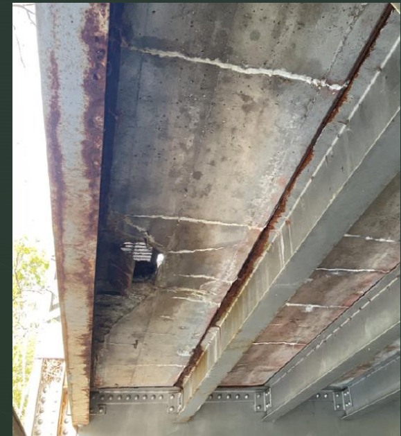
Typical Deck Cracking.
