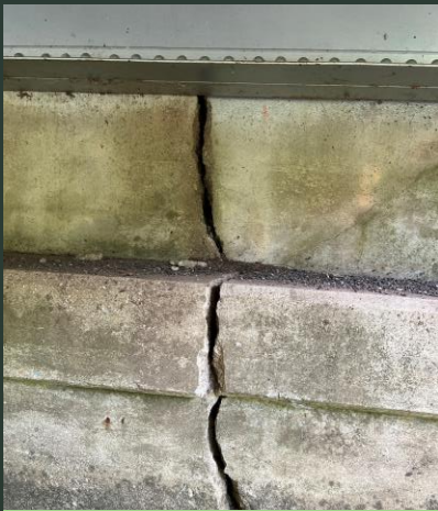
East Abutment – Vertical Crack.
